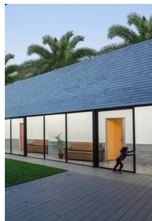
Figura 77 Patio central. Fuente: Archdaily.
