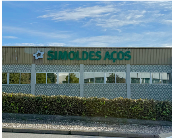
Figure 1. Exterior view of Simoldes Aços, located in Oliveira de Azeméis, Portugal.
