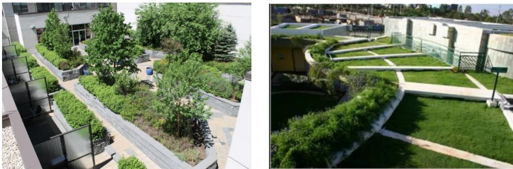
Figure 2. Rooftop garden: intensive system (top) and extensive system (below)
