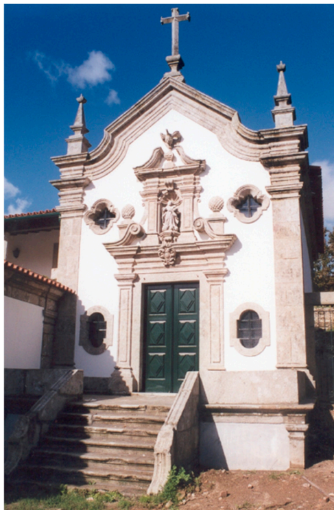
Figure 9. Nossa Senhora do Rosário Chapel in Linhares. Source: authors.
