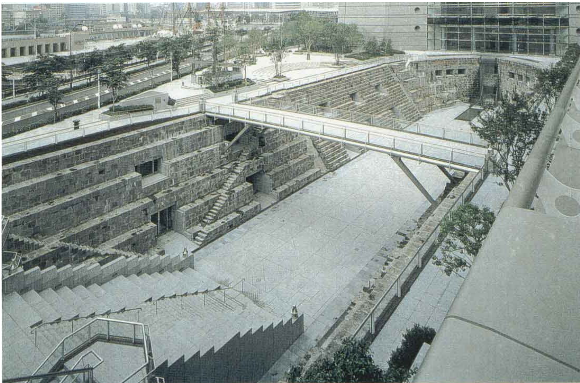
17. Photographs taken before and after the intervention. Several windows, a transversal bridge, staircases, are some of the elements that were used to transform the original Dry Dock #2
