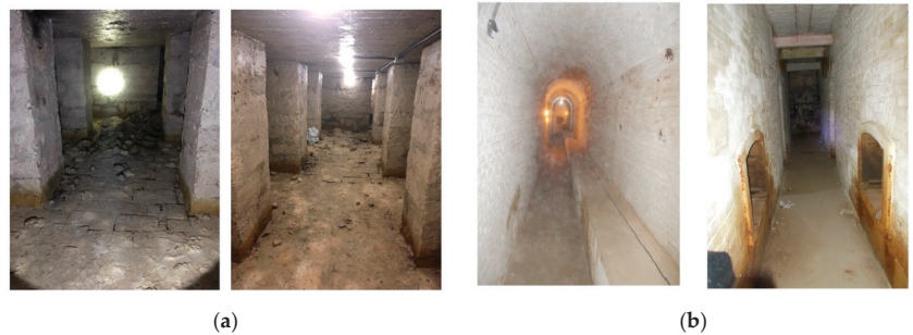
Figure 1. Air-raid shelters in the EDUSI area: (a) photographs of the interior of the R35 Marva Promenade shelter; (b) photographs of the interior of the R69 Tobacco Factory shelter. Own work.
