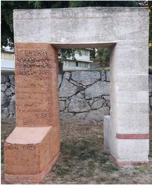
FIGURE 5 The Rammed Earth Portico on the University of Minho campus, used in the case study.
