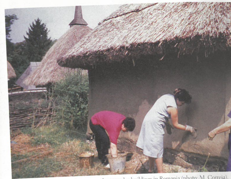
Fig. 12 Communitarian maintenance of vernacular buildings in Romania (photo: M. Correia).
