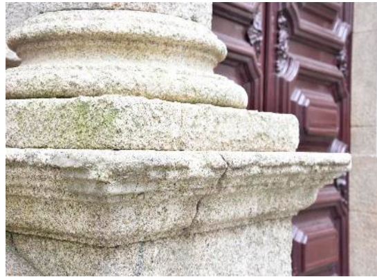
Figure 30. Identification of the various pathologies on the north façade of Vitória Church, Porto. Source: Author.
