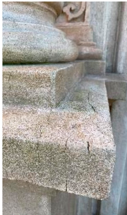
Figure 21. Identification of the various pathologies on the north facade of São João Novo Church. Source: Author.
