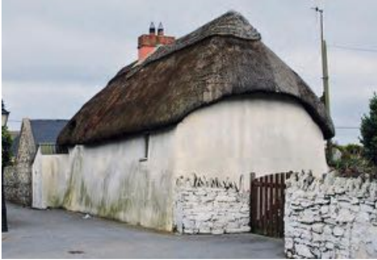
Mud house, plastered with cement / Kilmore Kay, Co. Wexford. The mud house of an old farm / Poulwitch, Mayglass, Co. Wexford. Two storeys mud house, plastered with cement / Next to Kilmore Quay, Co. Wexford. (photos: Marie Chabenat)
