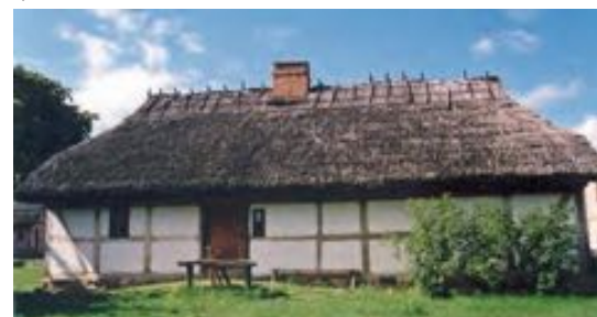
Half timber cottage (XIX c) with wattle and daub in fill, in Nadole, Pomorze. (photo: Teresa Kelm)
