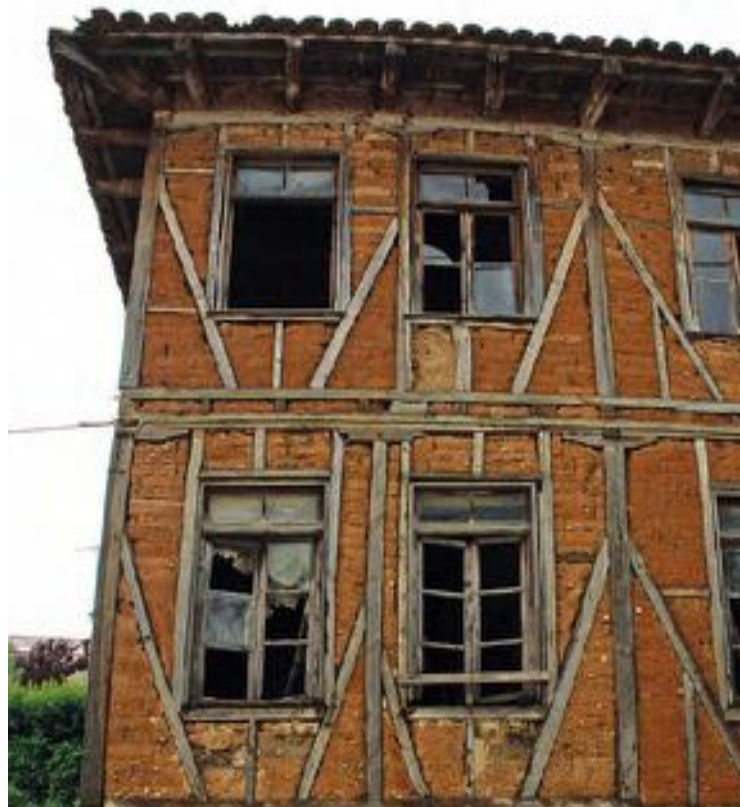
Traditional buildings in Kastaneri. (photo: Saverio Mecca) Sahnissi (architectural projection) made of tsatma. Village Paleos Panteleimon, prefecture of Pieria.
