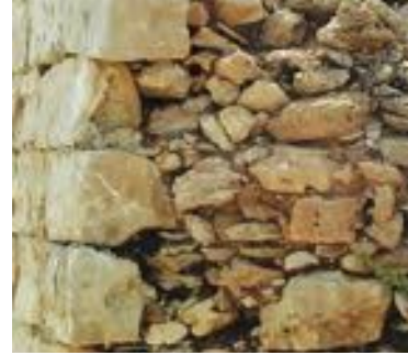
Wall with earthen mortar in Malta. (photos: Maria Mifsud)
