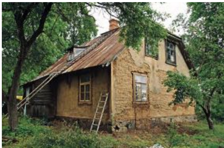
Rammed earth dwelling house built in 1926. The facade after the removal of damaged parts of the old plaster. Rēzekne district, Viļāni parish. (photos P. Blūms)
