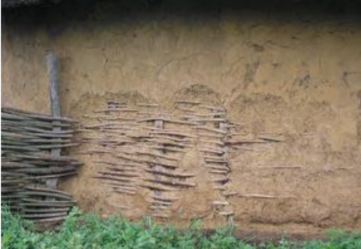
Detail of the exterior walls, Museum Debjerg Jernalder, in Skjern. (photos: Jacob Merten) Construction site for compressed earth blocks (CEB), by OSKAM company, in Kolind.
