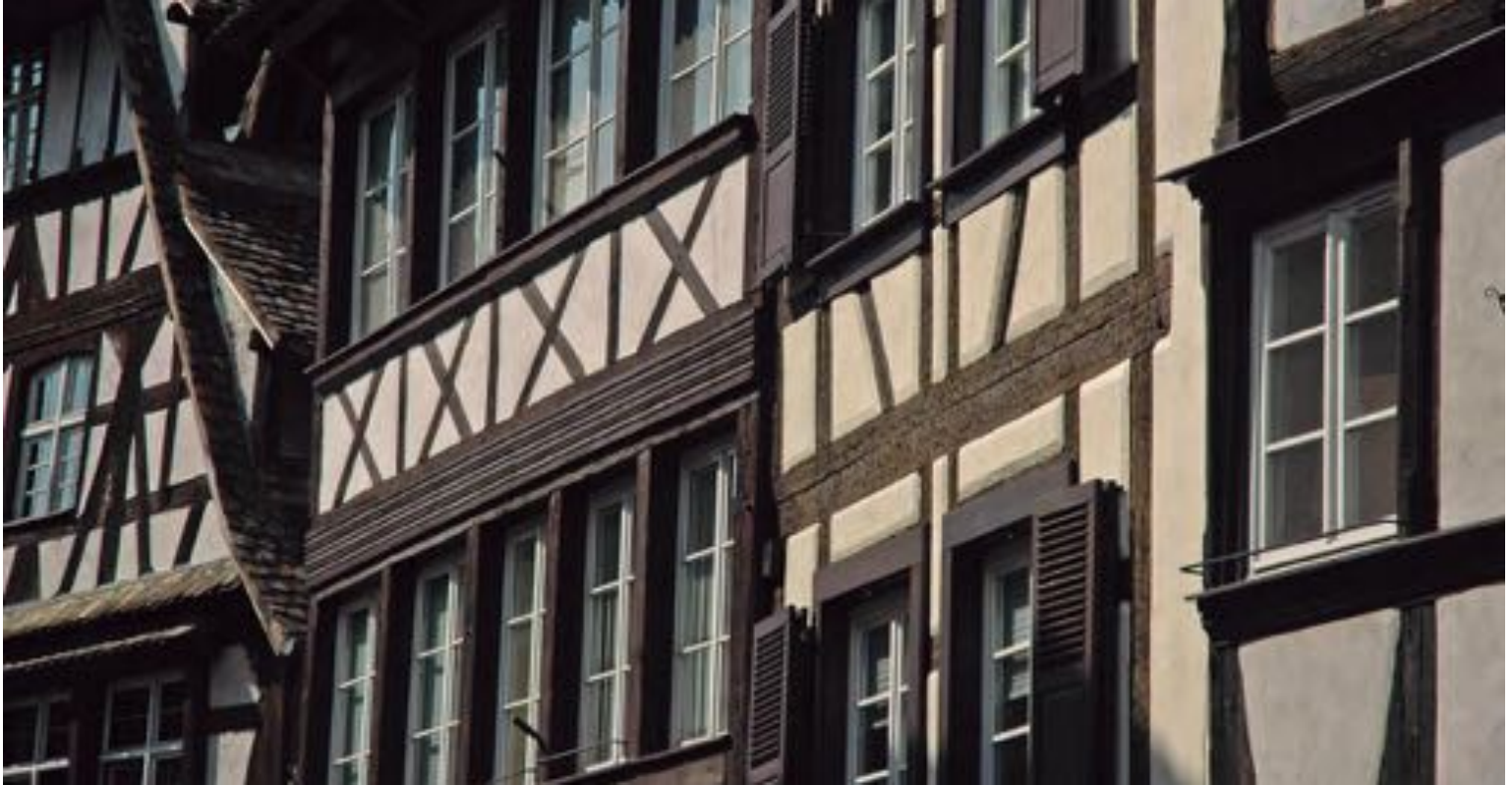
Timber-framed houses, formerly filled with wattle and daub, now with current materials: bricks or cellular concrete, Alsace, France. (photo from Terra Incognita. Discovering/Preserving European earthen architecture , Argumentum/Culture Lab Editions, 2008)
