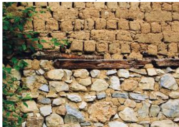
Stone basement and adobe wall in the region of Gotse Delchev. (photo: Saverio Mecca)
