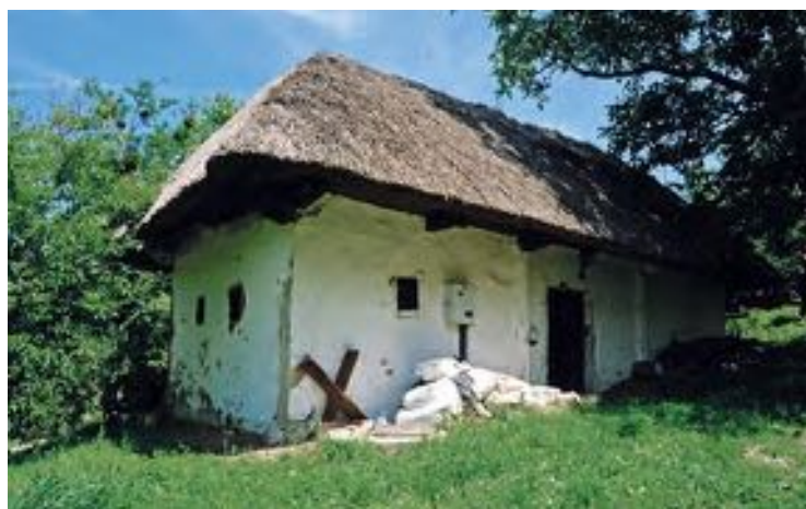
Wooden construction wine cellar. The cellar is under the living room, called the 'hisa' (Penova kleit, Filovski gaj) (photos: Borut Juvanec)
