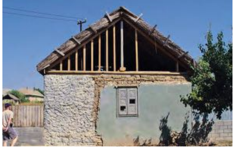
House under renovation in Dobrogea region
