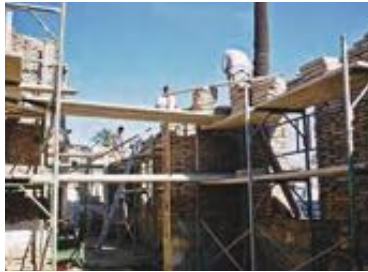
Use of adobe bricks in the restoration of the Museums of the Pancyprian Gymnasium, Nicosia, Cyprus.
