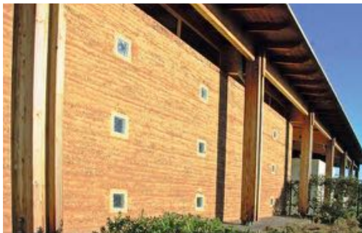
Social housing "Le Village" (1998-2009), CEB walls, Cavailon, Vaucluse. (photo: René Guérin)
