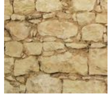
Wall with earthen mortar in Malta. (photos: Maria Mifsud)
