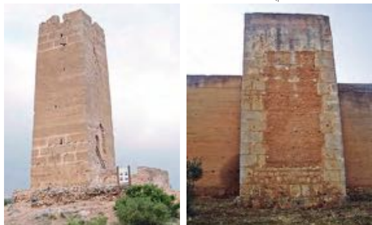
Example of reinforced earth wall with lime and stones, Bofilla tower, Bétera, Valencia, Comunidad Valenciana. (photo: Fernando Vegas with Camilla Mileto) Example of tapia calicestrada wall, city wall of Niebla, Huelva, Andalucía. (photo: Valentina Cristini)
