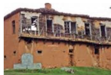
Two storeys adobe building in Kastaneri village. (photo: Saverio Mecca) Three storeys adobe building in Kranionas village, municipality of Kastoria. Sahnissi made of tsatma . Ano Kranionas village, municipality of Kastoria. Connection between ground and first floor by internal staircase leading to loggia. Ano Kranionas village, municipality of Kastoria. (photos: Georgia Bei)
