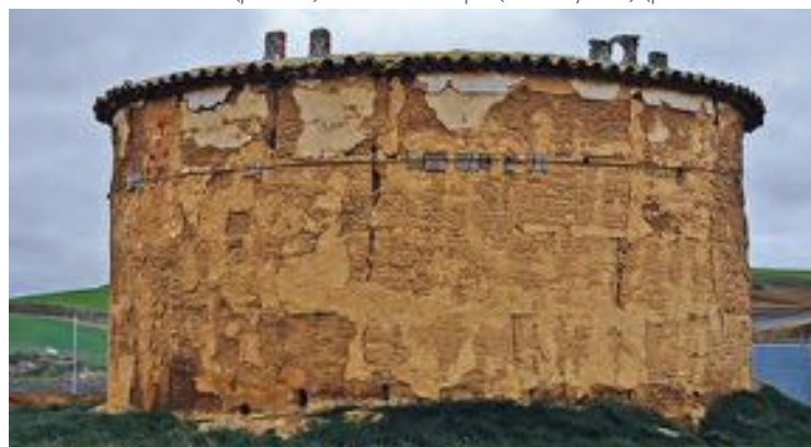
Example of reinforced earth wall with lime and stones, Bofilla tower, Bétera, Valencia, Comunidad Valenciana. (photo: Fernando Vegas with Camilla Mileto) Example of tapia calicestrada wall, city wall of Niebla, Huelva, Andalucía. (photo: Valentina Cristini)
