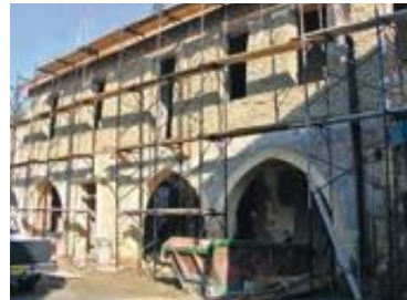
Adobe residence during its restoration
