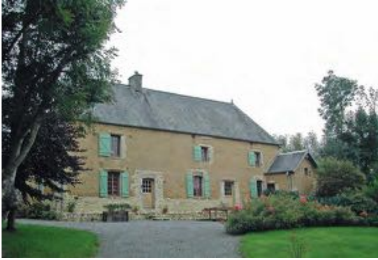
Cob house, Cotentin, Normandy, France. (photo from Terra Incognita. Discovering/Preserving European earthen architecture , Argumentum/Culture Lab Editions, 2008)
