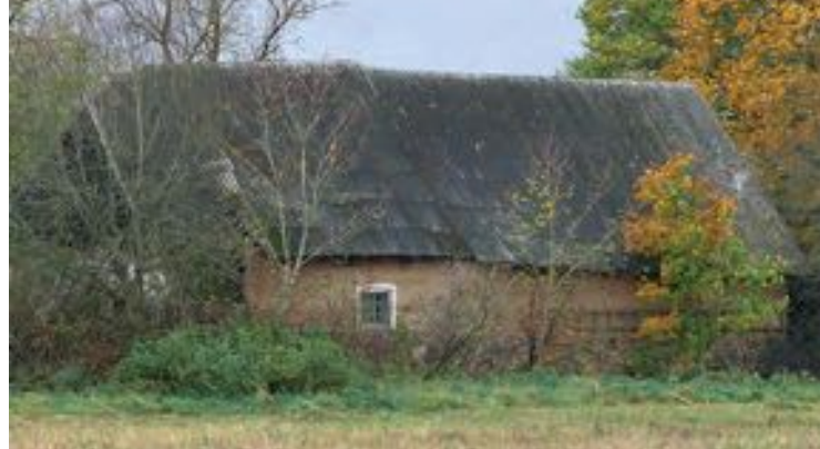
Barn in rammed earth in Tatumaa. (photo: René Guérin)
