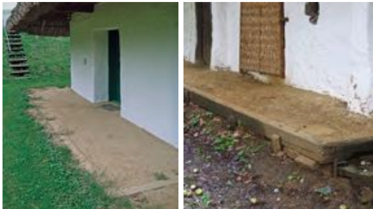
Exterior sidewalk enclosed by timber under thatched eaves in Heiligenbrunn Village. Rammed earth sidewalk enclosed by timber. Traditional house in Heiligenbrunn Village. Reconstruction of the interior space of an earthen house, Gerersdorf Open Air Museum. (photos: Fernando Vegas, Camilla Mileto)
