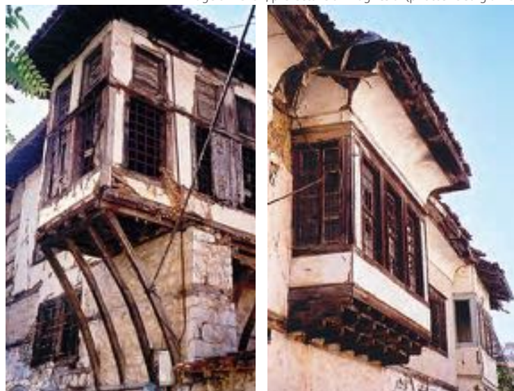
Adobe walls and Sahnissi on the upper floor. Agios Lavrelios, village of Pelion, prefecture of Magnesia. (photos: Georgia Bei)
