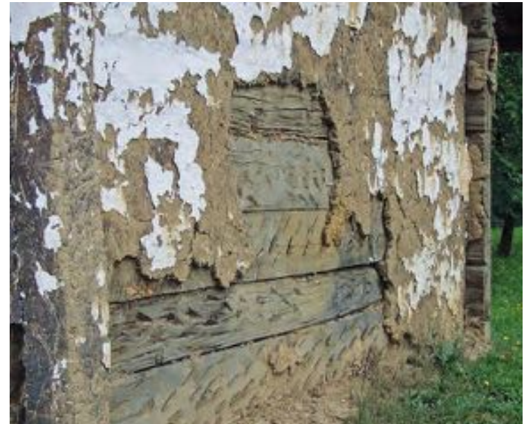
Earth coating detail, partially detached. Logslice house in Heiligenbrünn Village. (photo: Fernando Vegas, Camilla Mileto)
