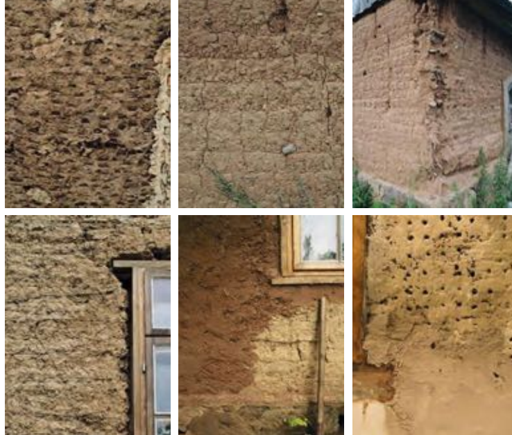
Rammed earth wall construction with fragments of broken ceramic roof tiles. Economy building of Bērzgale manor. Rēzekne district, Bērzgale parish.
