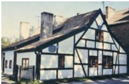
Half timber house with adobe masonry in fill (XVII c.), in Hel, Pomorze. (photo: Teresa Kelm)
