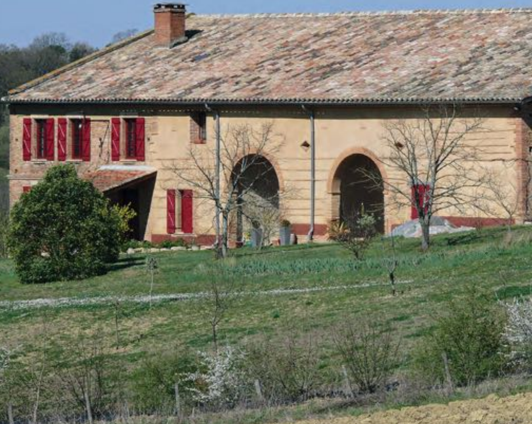
Farmhouse in rammed earth, adobe and bricks in La Salvétat-Belmontet, Tarn-et-Garonne. (photo: René Guérin)
