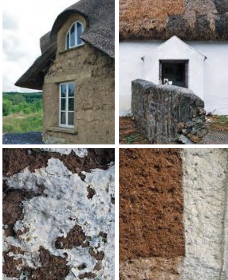
Contemporary mud house (self built) / Owing, Co. Kilkenny. The mud house of an old farm / Poulwitch, Mayglass, Co. Wexford. Farm building/ Limewashes detail / Effin, Kilmallock, Co. Limerick. Sample of lime plasters on clay walls / Traditional Lime Company / Tullow, Co. Carlow. (photos: Marie Chabenat)
