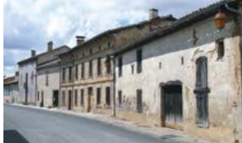
Adobe houses, Salvagnac, Tarn. (photo: René Guérin)
