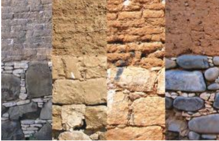
Adobe masonry constructed on a stone foundation: Ayia Varvara; Nicosia; Limassol and Orounta
