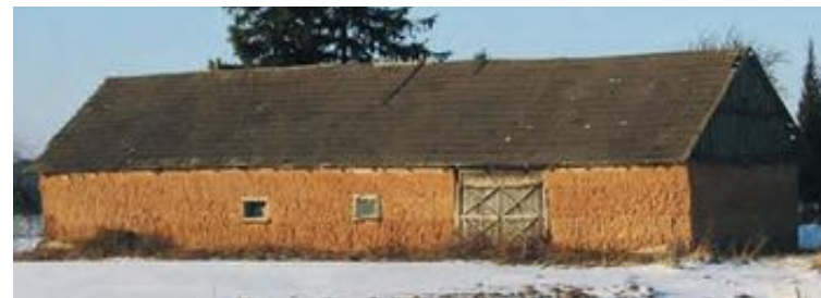
Non-plastered out-house, made with clay, Rokiškis district.
