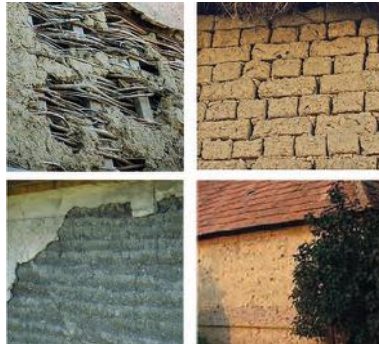
Different types of earthen techniques observed in Slovakia. (photos: Boris Hochel, Zuzana Kierulfová and Inez Búci)
