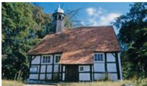
Church (XVIII c) in adobe masonry, in Wytowno, Pomorze. (photo: Teresa Kelm)
