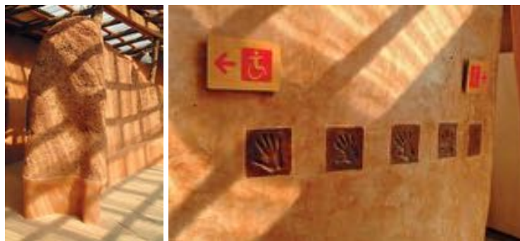
Modern cob building, Jackie Abey and Jill Smallcombe, Eden Visitor Centre, Cornwall, UK. (photos: Louise Cooke)
