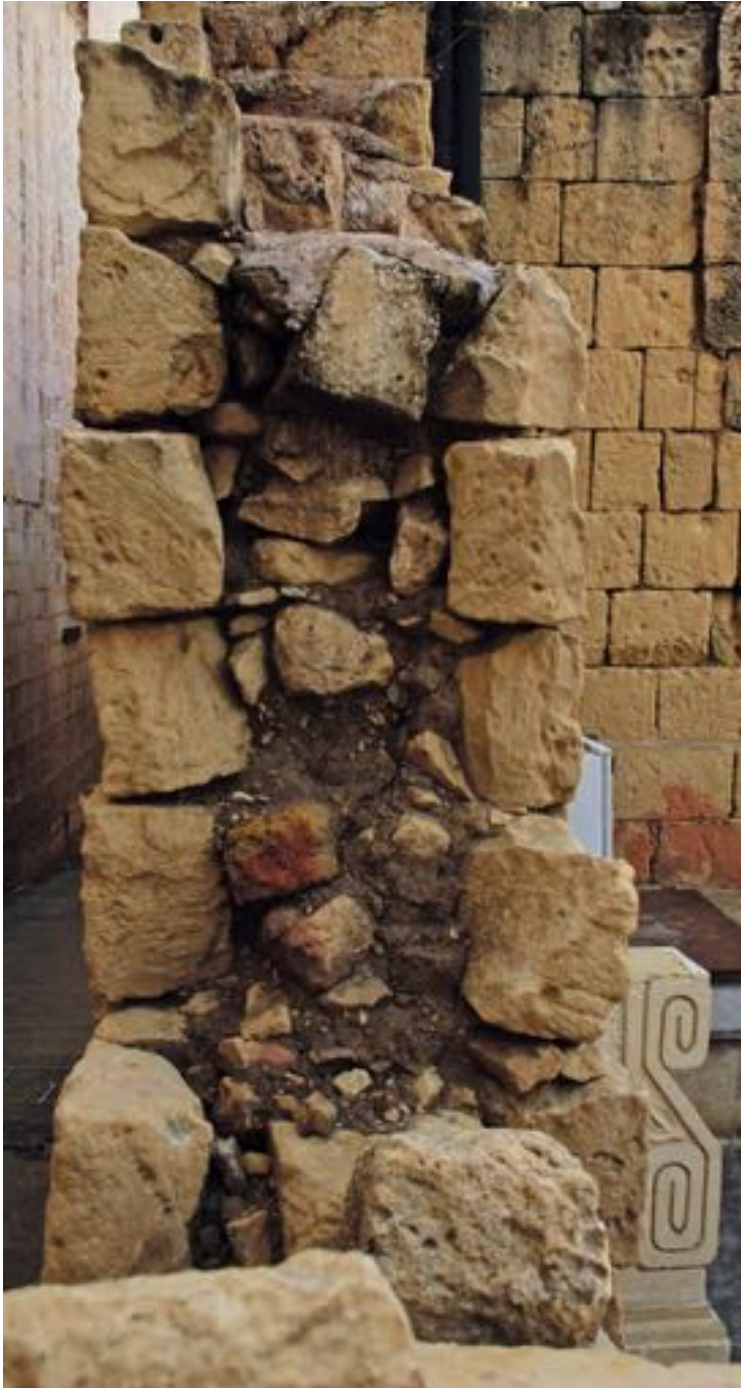
Wall with earthen mortar in Malta. (photos: Maria Mifsud)
