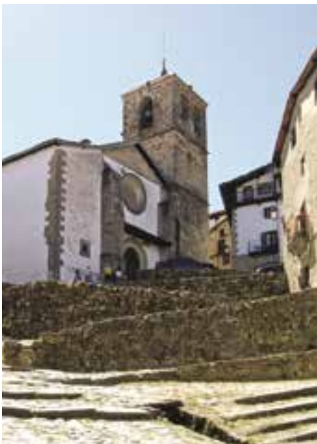
Fig. 6: Channels drains ( regaderas ) along the streets in Candelario, Spain (photo: M. Cadinu).
