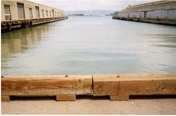
10. Deck and pier were removed to free the view
