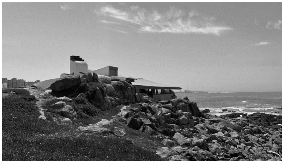
Figure 4. Tea House—North View—2023. Reproduced with permission from Susana Milão, Photo_CIAUD-UPT, author archive, 2023.
