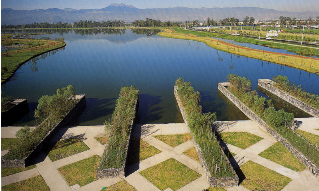
3. Xochimilco Ecological Park, Mexico City, Grupo de Diseño Urbano, 1993 View of the pumping system .
