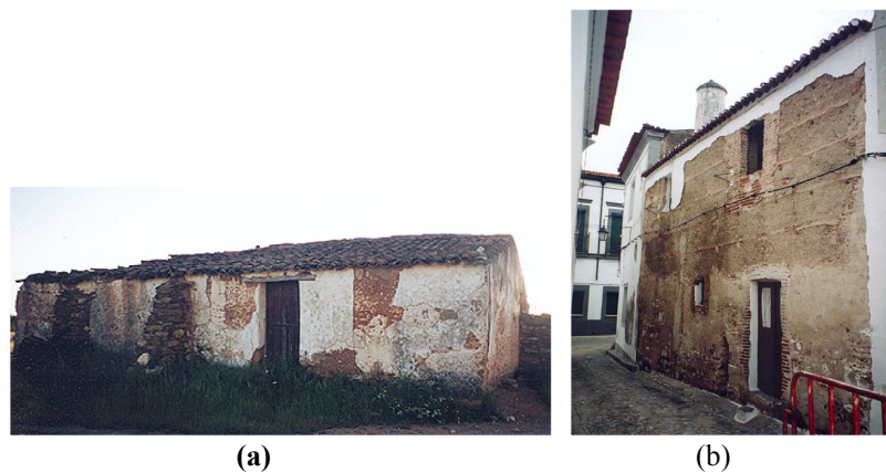
Figure 3. (a) Traditional rural one-floor rammed earth vernacular construction in Alentejo, Portugal (Correia 2007); and (b) traditional urban two-floor rammed earth construction in Alentejo, Portugal (Correia 2002)
