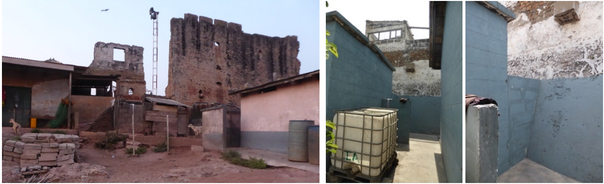
Figs. 30 to 32 – Illegal construction was built around Fort Nassau (fig.30), and Fort Prinzenstein (figs.31 & 32).
