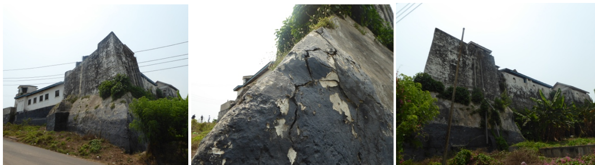
Figs. 181 to 183 – The rising of vegetation that is growing in the façades brought additional problems to the structure.
