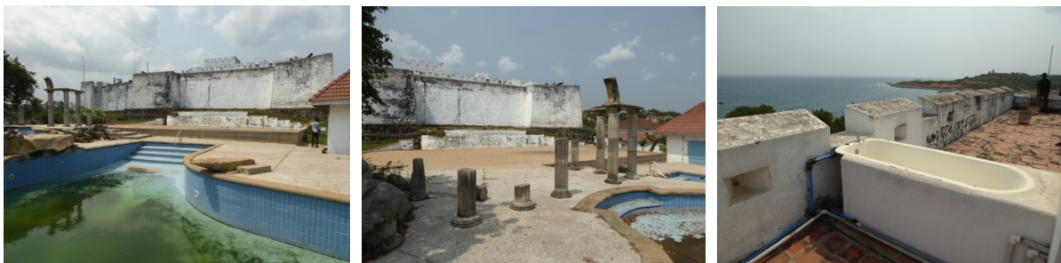
Figs. 25 to 27 – A swimming pool, roman style cement columns, and a bath tube were built in and around Metal Cross Fort.
