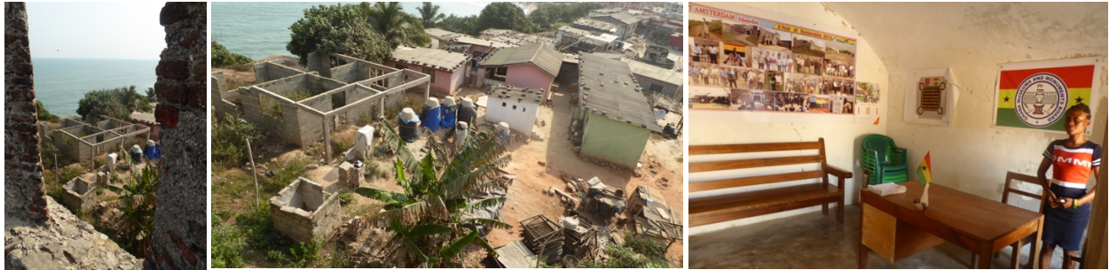
Figs. 105 to 107 – Encroachment and urban pressure continues to grow near the fort. Visitor centre in one of the fort rooms.
