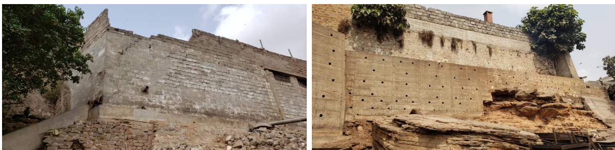
Figs. 28 & 29 – Cement bricks were added to the walls of Fort James.
