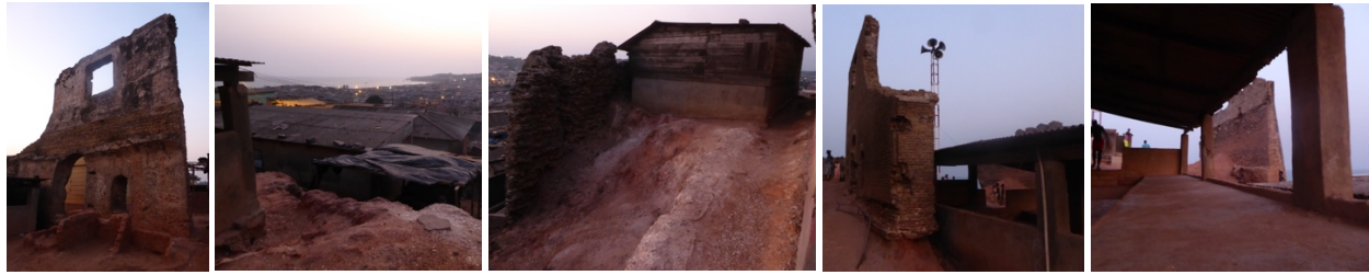
Figs. 115 to 119 – View of the remain walls still standing in Fort Nassau (fig.115), urban pressure (fig.116), encroachment (fig.117), and a new concrete religious building that was erected touching the last remains of the fort archaeological walls (figs.118 & 119).
