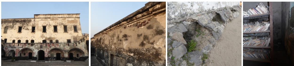
Figs. 108 to 111 – Interior terrace at Fort William (fig.108), inadequate cement plasters (fig.109), impact of the sea erosion in the East side of the building (fig.110), and abandoned library at the fort (fig.111).
