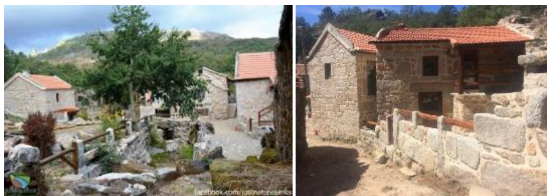
Figure 7. The winter village of Pontes and its central cluster of houses (credit: Justnature). Photo at right shows buildings under retrofitting at the time of the workshop.
