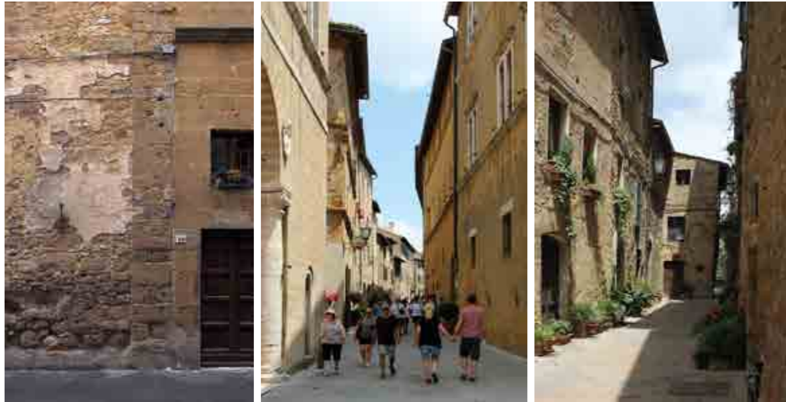
↑ Images of the deterioration in building facades
