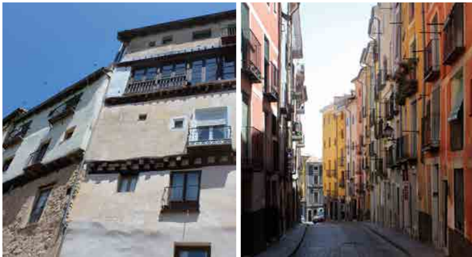
↑ Facades still conserving constructive features of traditional architecture from Cuenca (© F. Vegas, C. Mileto, 2017)
